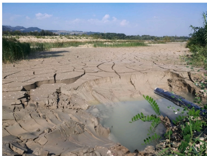
Fig. 2. Silt collection and settling areas at the S.A.P.A.B.A. landfill site, Italy.
