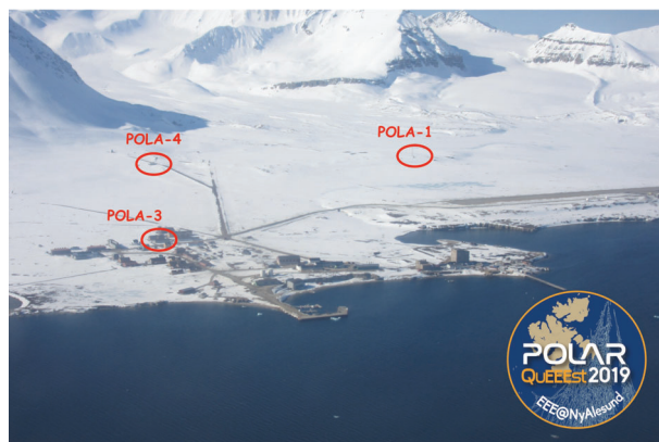
Figure 1. Aerial photo of Ny Ålesund, 79°N in the Svalbard archipelago. The red circles indicate the installation sites of the POLA-R detectors, inside buildings managed by the Italian CNR: POLA-1 in the hutch of the Climate Change Tower, POLA-3 inside the Dirigibile-Italia Base and POLA-4 in the Gruvebadet Laboratory.
