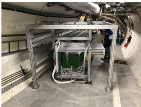
Figure 2. Installed aluminium frame
