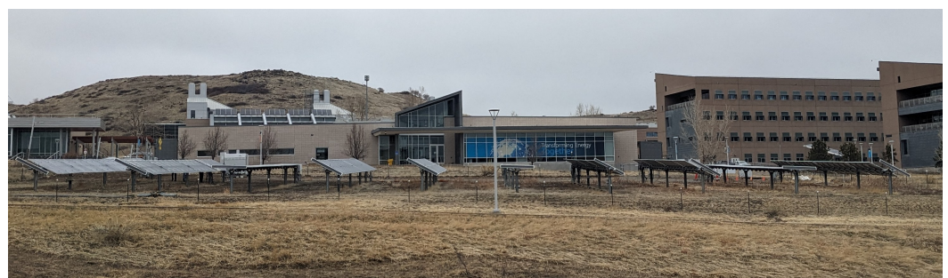
Figure 2. Picture of the PV field during an overcast day (7th of March 2025). It can be seen how some rows are fixed at 0^\circ while the others are tracking.
