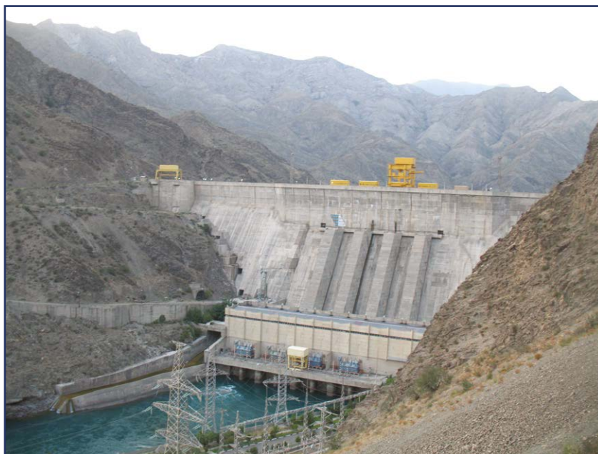
Fig. 14.9. Kürpsay hydroelectric dam in Kyrgyzstan. Image: Wikimedia/Firespeaker.
