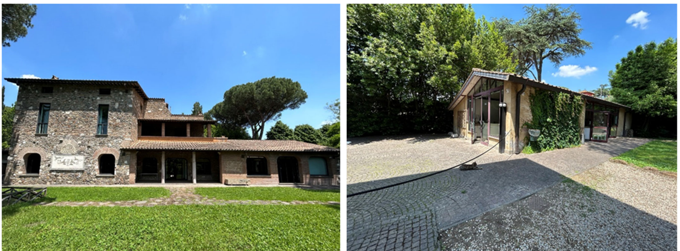
Figure 5. The Capo di Bove complex: main building, on the left, and outbuilding, on the right.
