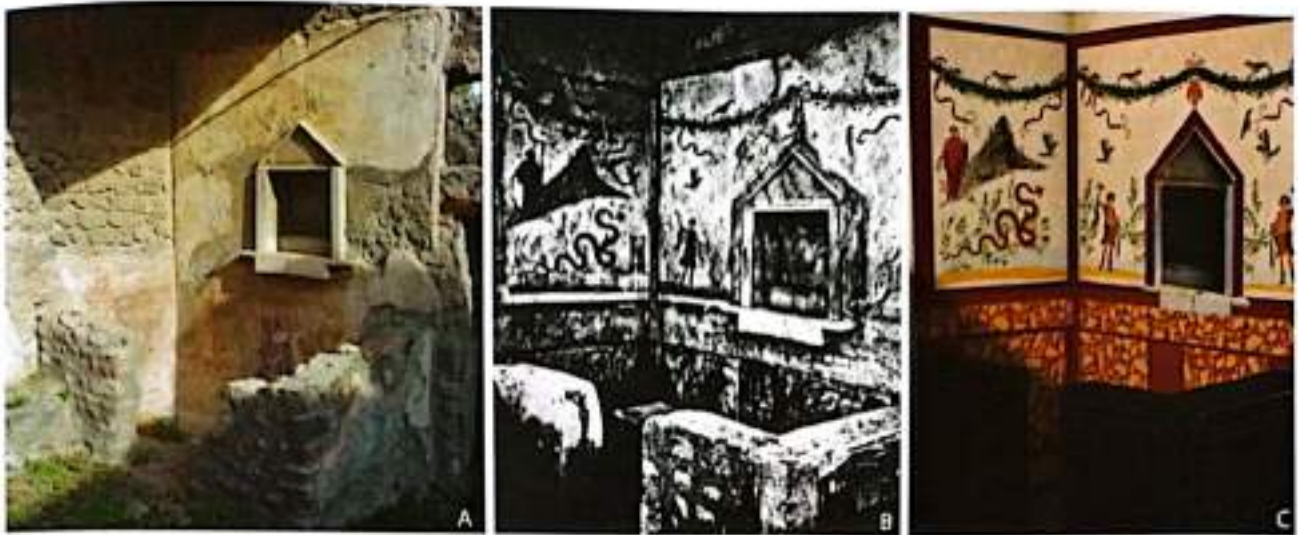
Fig. 9: Pompeii. Insula IX 8, Casa del Centenario (IX 8, 3.6.a), small atrium (49), lararium. A: current situation. B: state of the early 20 th century. C: virtual restoration.
