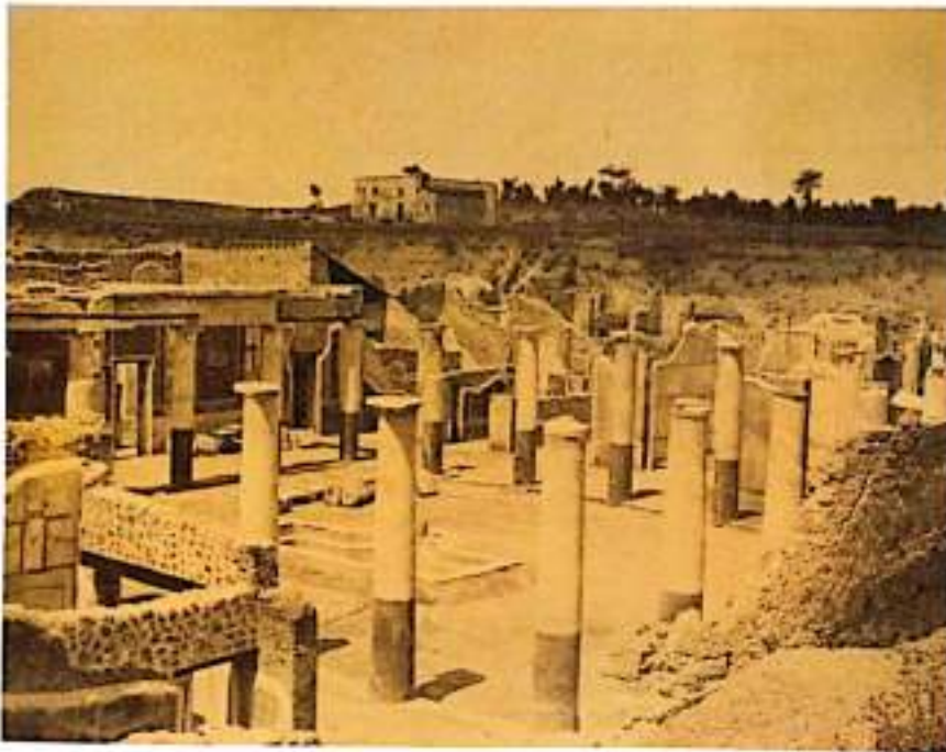
Fig. 5a: Pompeii, Insula IX 8, Casa del Centenario (IX 8, 3.6.a), peristylum 9, from south-east: excavations in progress (at the right, the eruptive deposits) and the first restoration measures.
