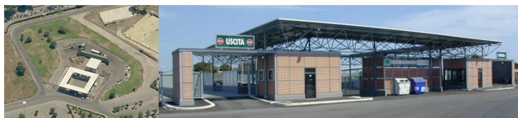
Figure 2. Ecological island, waste collection center, Rome, Italy.
