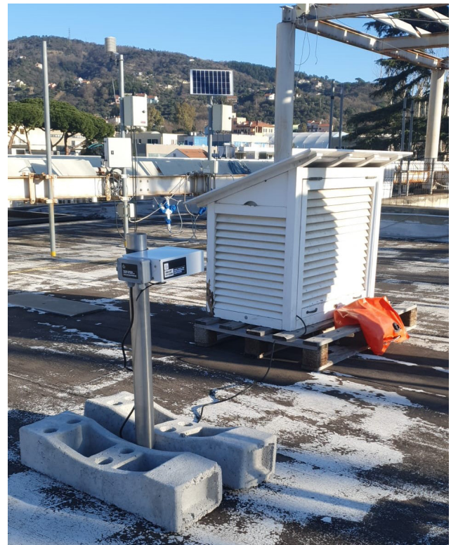
Figure 3. Stevenson screen (front right) and reference weather station (middle back) locations on the building rooftop.
