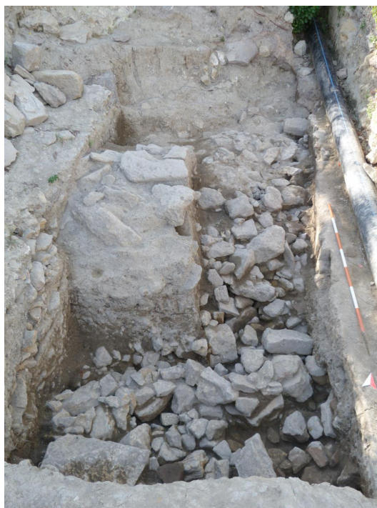
Fig. 5. Ghattarello (Ancona). Collapse of the circuit wall (trench 3).
