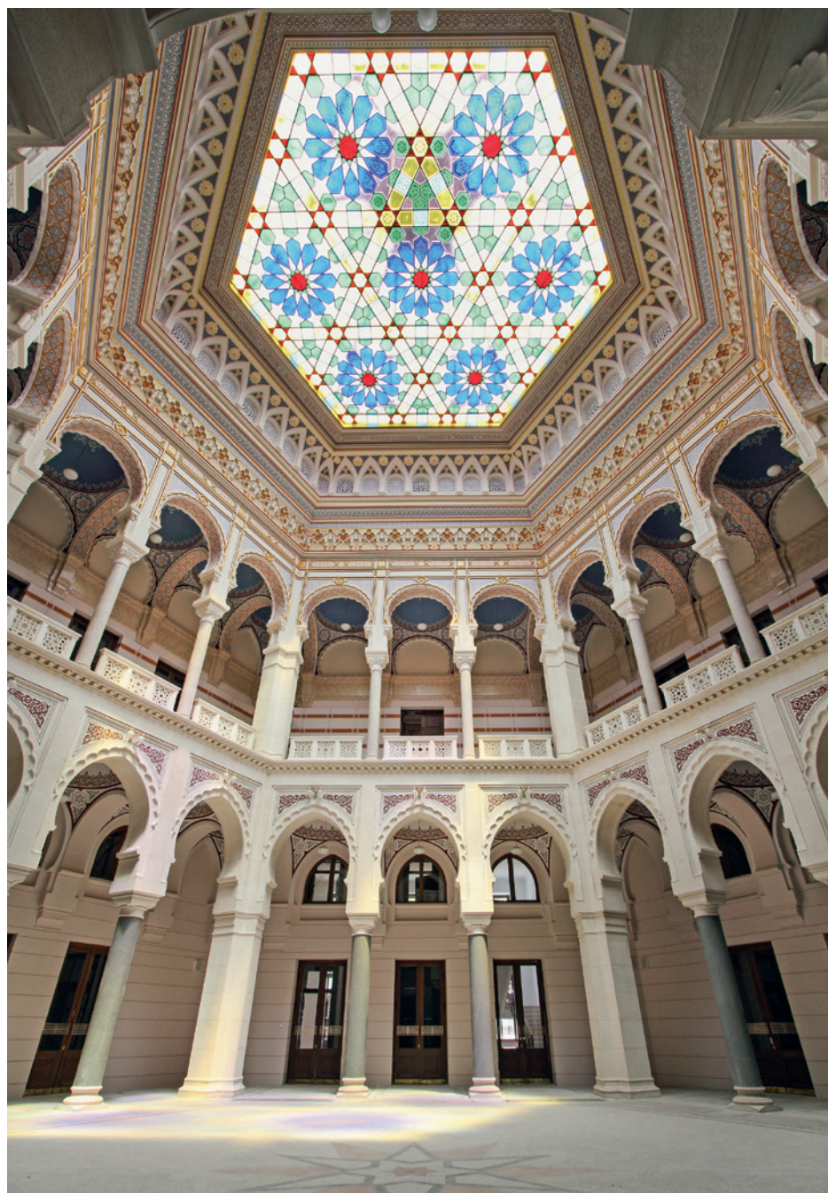
Fig. 12. The stained-glass roof of the hexagonal courtyard in the Vijećnica of Sarajevo (1892–95). Photograph by Anida Krečo.
