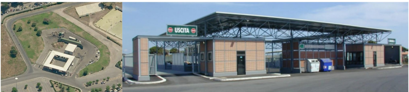
Fig. 1 Ecological island, waste collection center, Rome, Italy
