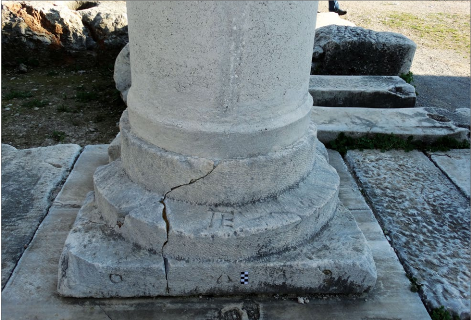
Fig. 7. Ephesos, basilica of St. John, column base with assembly/positioning and workshop marks (Photo G. Marsili)
