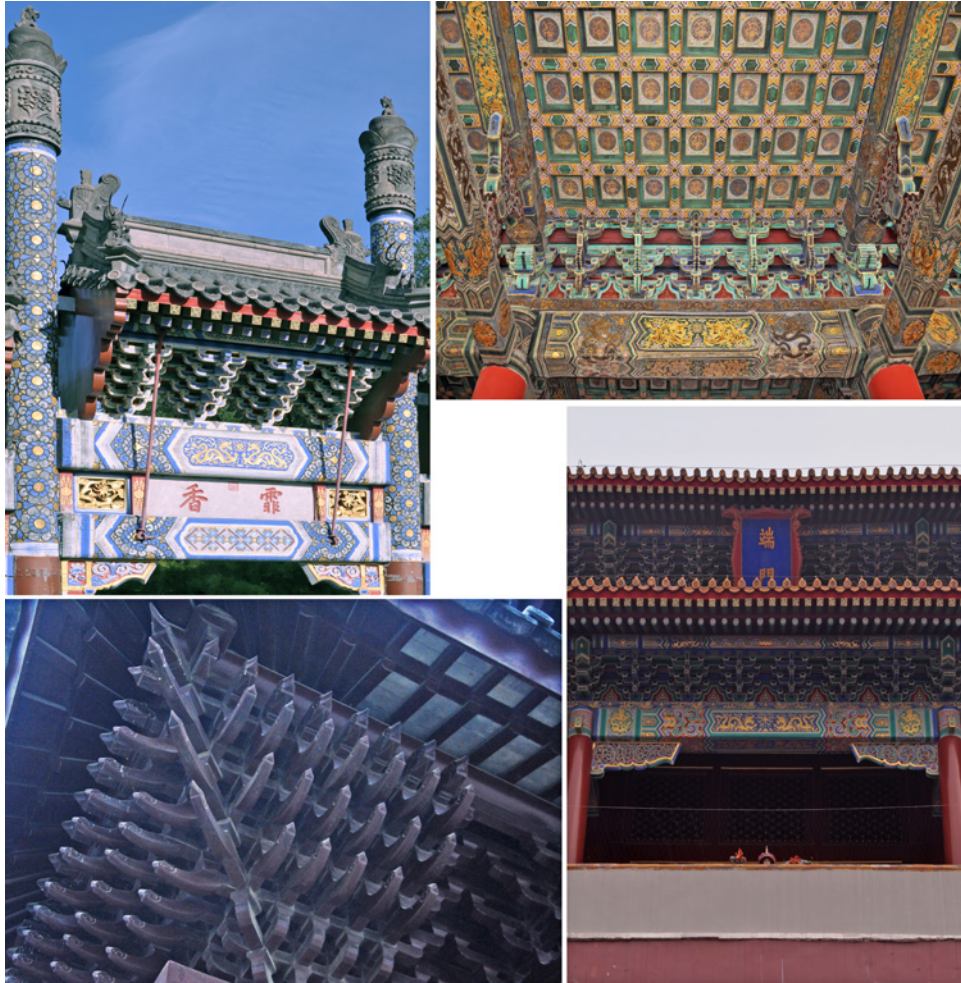
Fig. 4. Examples of different types of bracketing systems in traditional Chinese buildings located in Beijing and Shanghai © 2011, C. Mazzoli.
