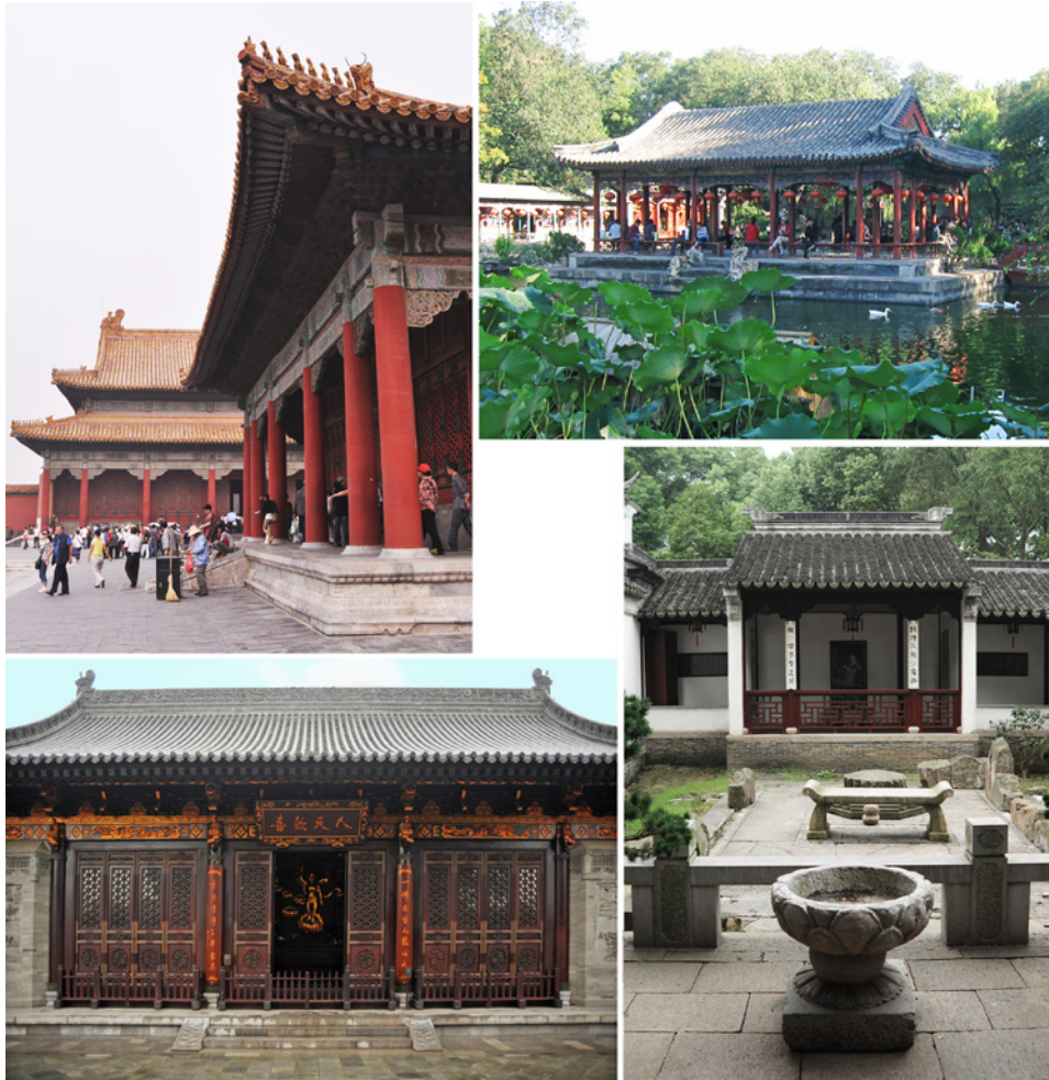
Fig. 3. Examples of stone foundations for traditional Chinese buildings located in Beijing, Shanghai, and Xi'an © 2011, C. Mazzoli.
