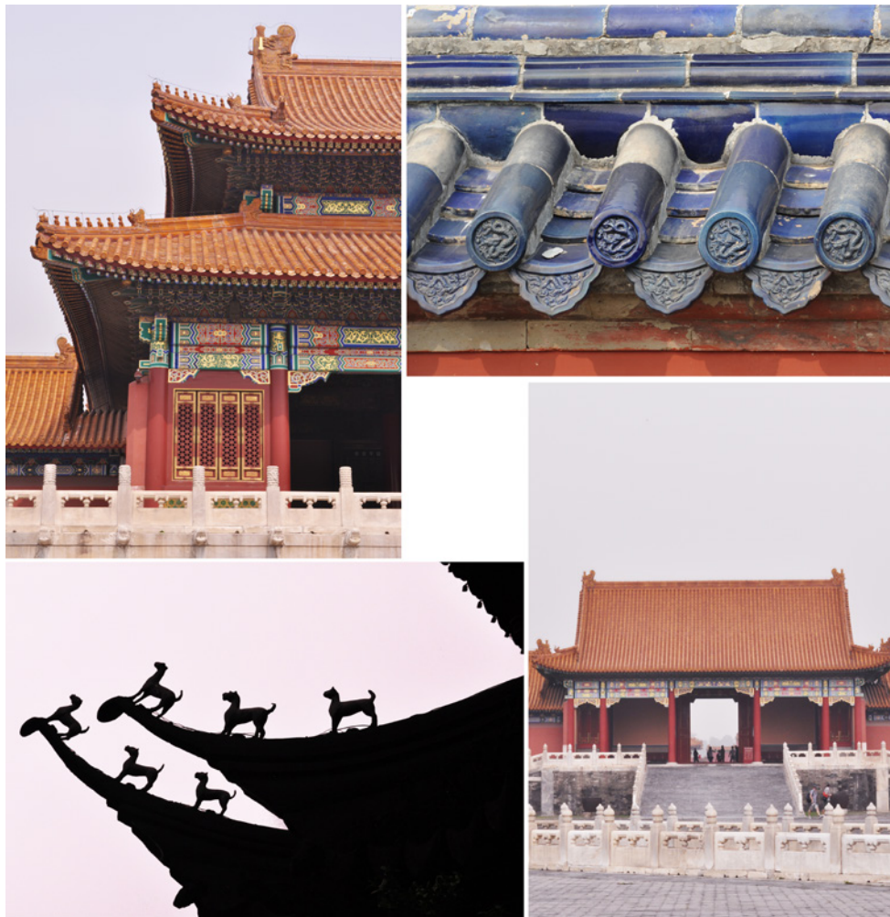
Fig. 8. Examples of different types of roofing systems in traditional Chinese religious buildings located in Beijing © 2011, C. Mazzoli.
