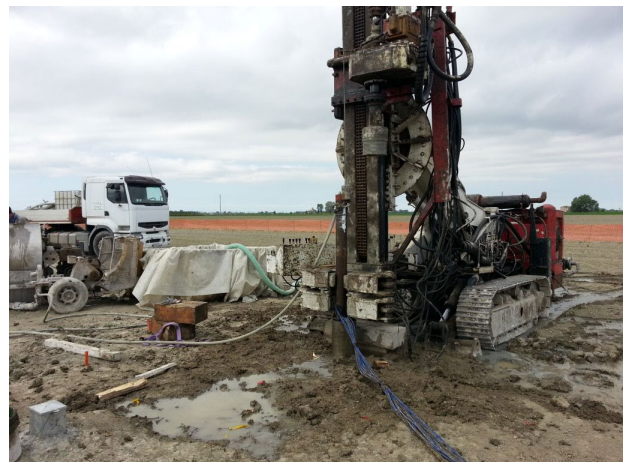
Figure 6. Installation of the instrumented micropile.
