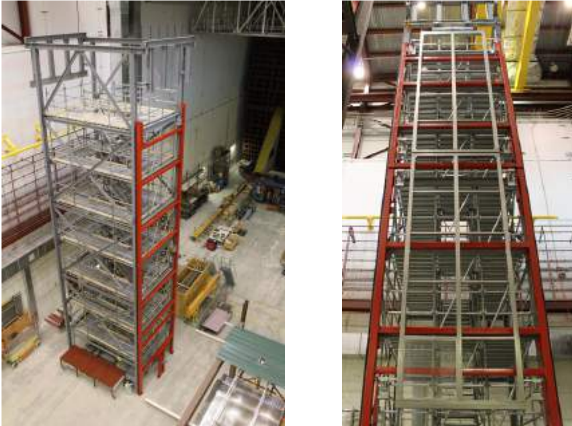
Figure 2.27. APA pair assembly and integration tests at Ash River.
