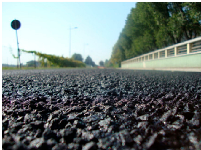
Figure 12. Cold laid acoustic microsurfacing at an Italian experimental site [69].
