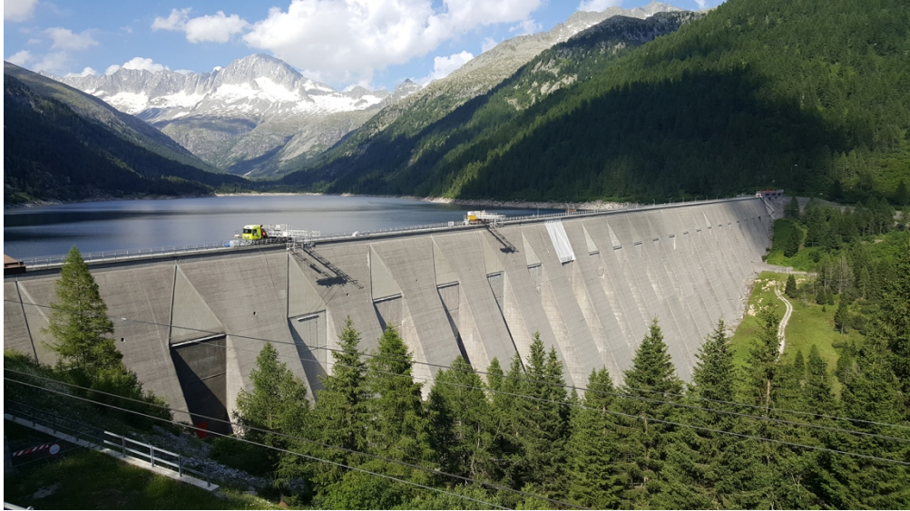
Figure 8. Cellular gravity dam (Marcello type) of Malga Bissina (photo taken by the authors on 05.07.2019).
