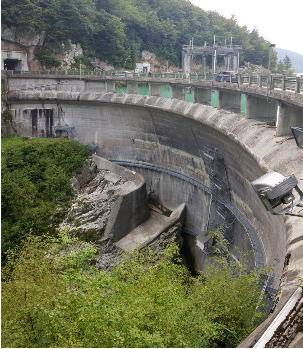
Figure 5. The double-curvature dam of Barcis (photo taken by the authors on 11.08.2019).
