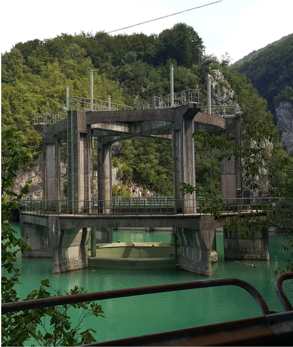
Figure 2. Intake structure of Barcis Dam (photo taken by the authors on 11.08.2019).
