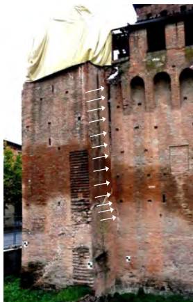
(a) N-E Tower - North wall joint: note the absence of connection between the parts
