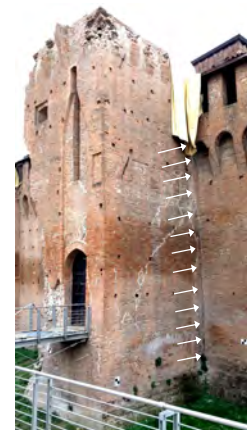
(c) North Tower - North wall joint: good quality connection
