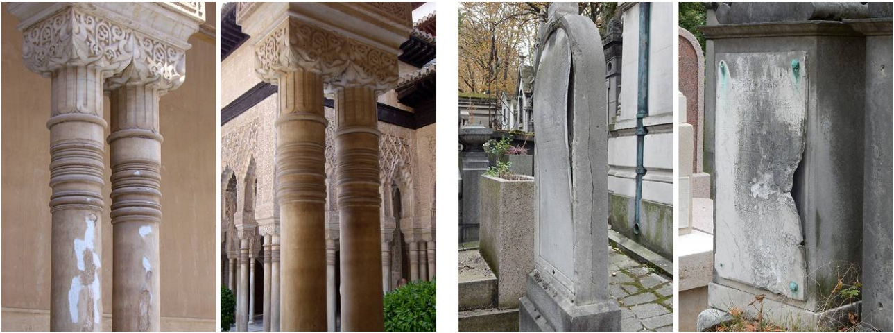
Figure 1. Examples of thermally induced degradation of marble. Left: Marble columns in the Courtyard of the Lions in the Alhambra of Granada (Spain, XIV century) exhibit severe granular disaggregation in the side directly exposed to solar radiation, while in the opposite sheltered side the same columns are substantially well preserved. Right: Thin slabs used as gravestones in the Père Lachaise Cemetery in Paris (France, XIX century) exhibit dramatic bowing and deformation.
