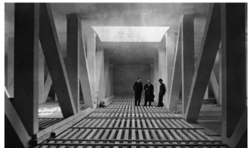
Figure 12. The roof skylight. Donati & Zanichelli Company's private archive.
