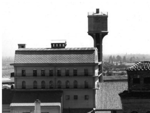
Figure 2. The stage tower and the piezometric tower in Bologna's landscape in 1935. Donati & Zanichelli Company's private archive.
