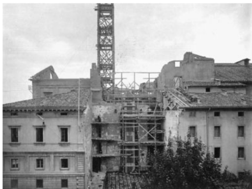
Figure 5. The reconstruction of the stage tower. Donati & Zanichelli Company's private archive.
