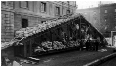
Figure 9. The load test of the metal beam. Donati & Zanichelli Company's private archive.
