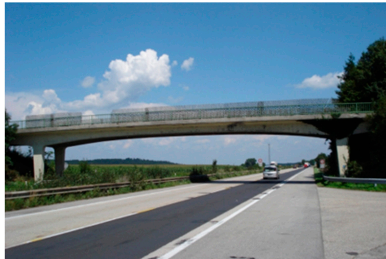
Figure 7. S101 bridge—West side [29].
