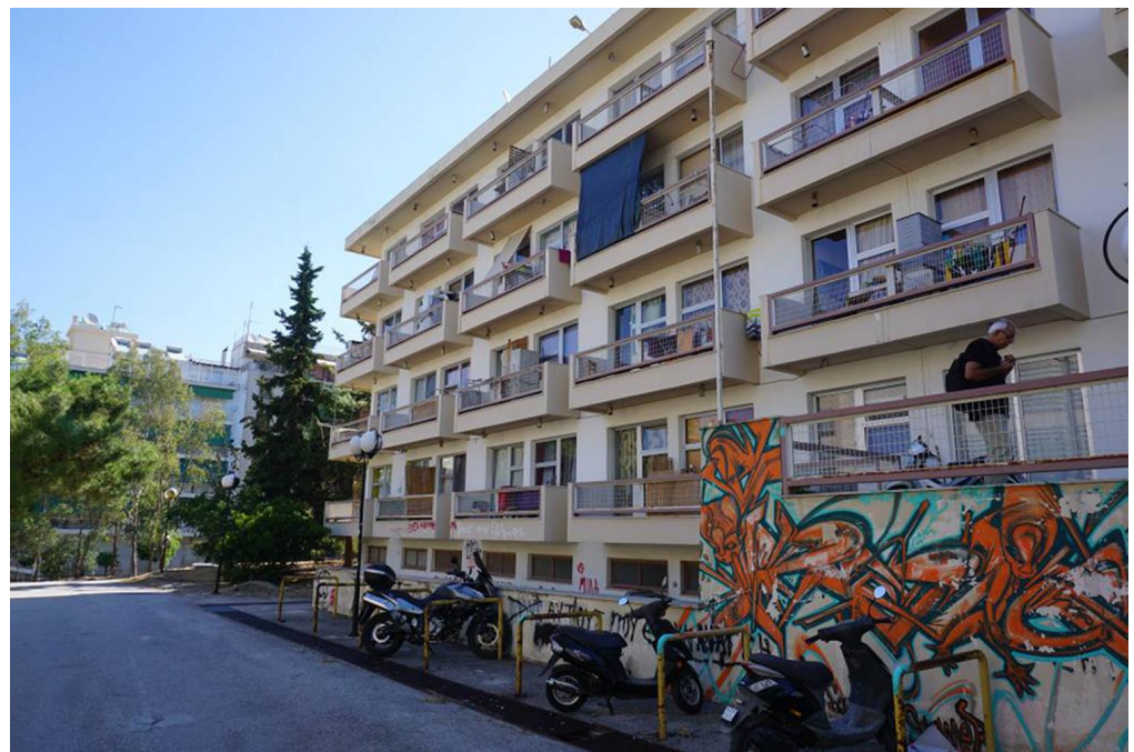
Figure 3. Student residence façade of the existing building. (© 2018, Authors).
