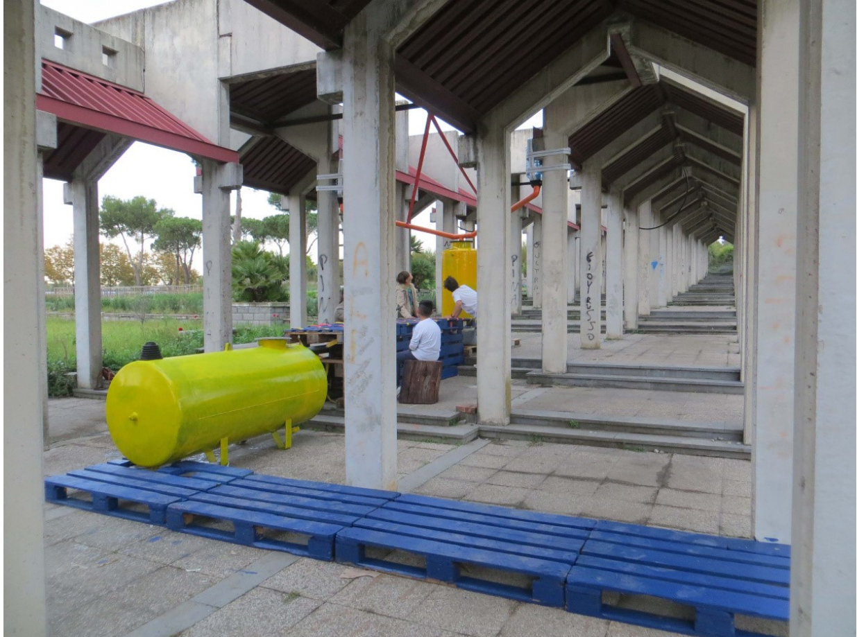
Figure 5: Self-built prototype for rainwater harvesting for irrigation realized with the repurpose of recycled materials in the Social Garden of Ponticelli.
