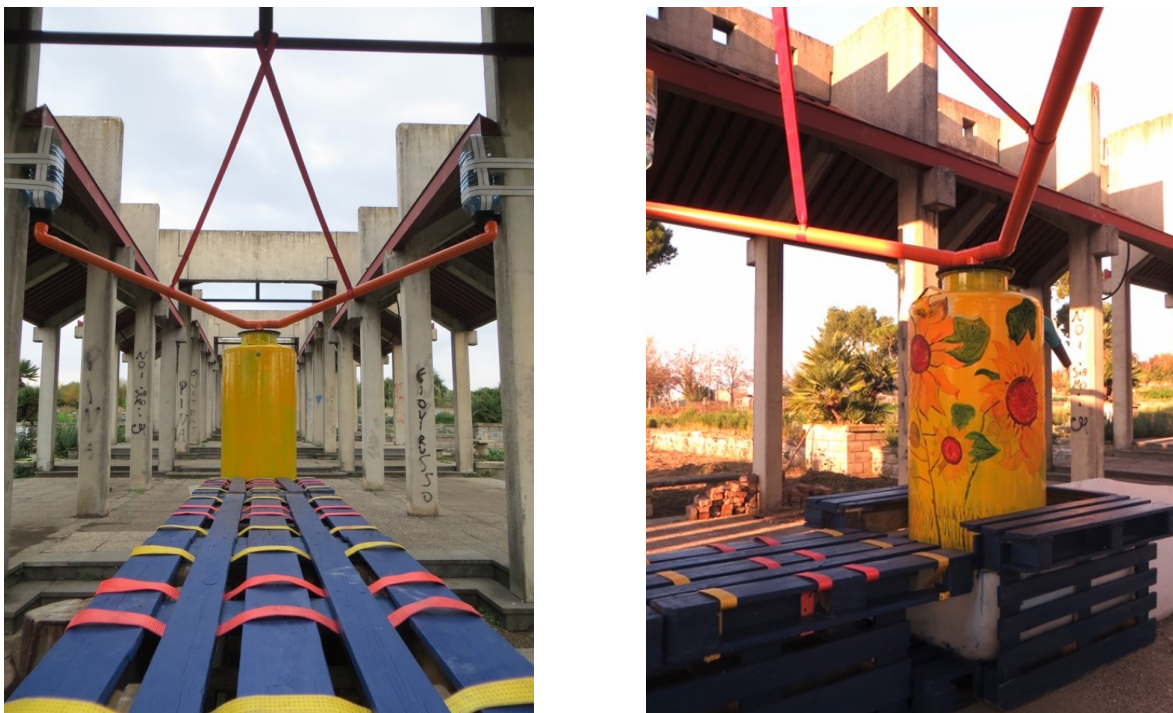
Figure 6: Prototype for the reuse of rainwater in the Social Garden of Ponticelli. The intervention was decorated by users.
