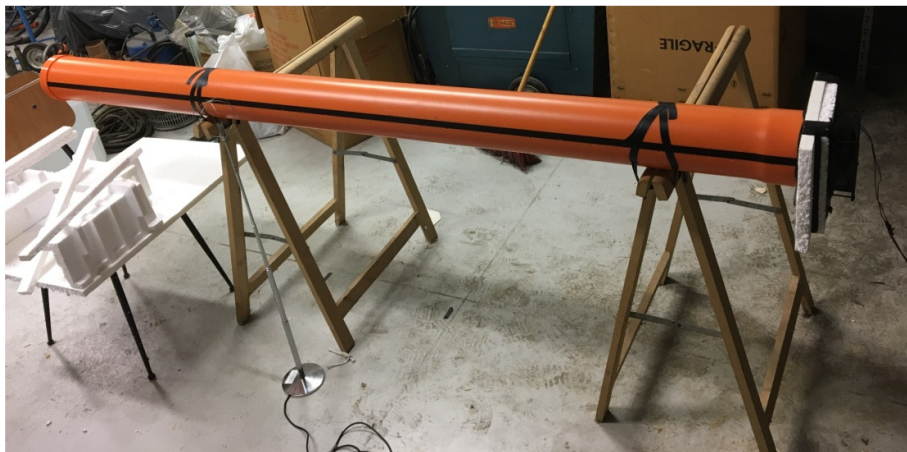
Figure 1. Micro ventilation system created for the cellar.
