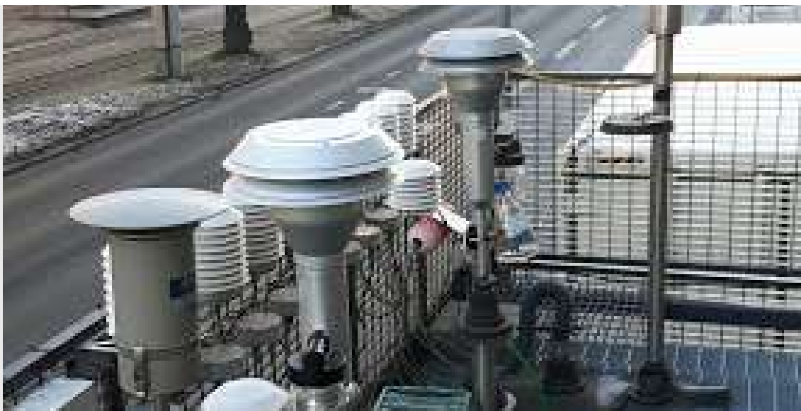
Fig. 29: Deployment of the Living Lab stations alongside the reference equipment at the operational air quality station of the Helsinki Region Environmental Services (HSY), November 2018, Helsinki (Finland). A larger-scale deployment with a similar set-up is planned in autumn 2019. Photo: Anssi Julkunen/HSY.
