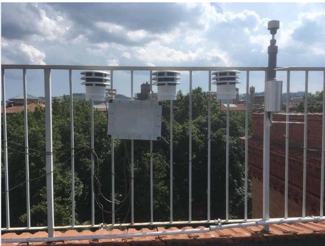
Fig. 15: Low-cost sensor deployment on the rooftop of the Department of Physics and Astronomy, UNIBO, June-July 2019, Bologna (Italy)
