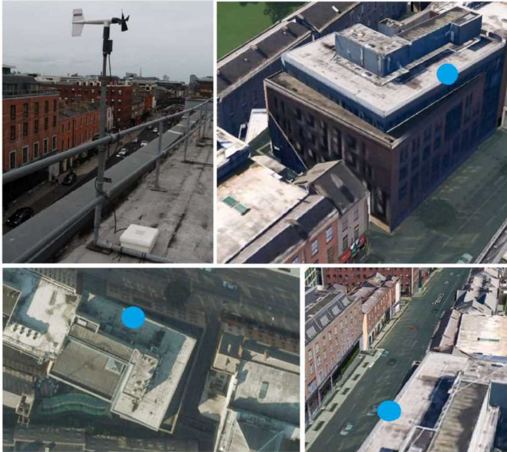
Figure 29: Wind Anemometer (Blue) on Pearse Street Rooftop.
