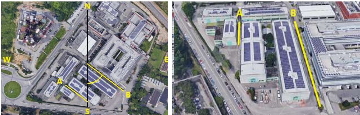
Figure 5: Overview of Lazzaretto site and surrounding area (left) and the two street canyons (right).
