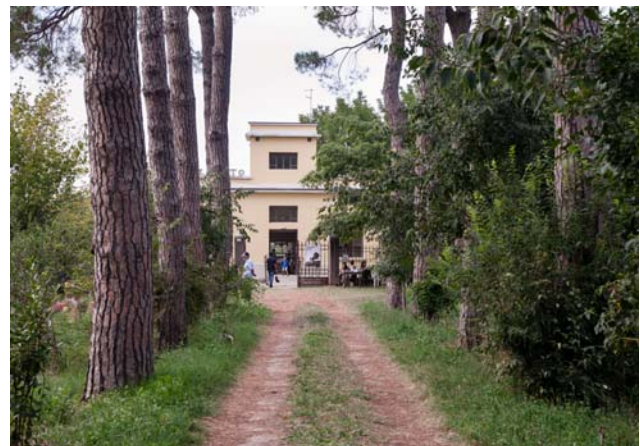
Fig. 9: The former Spinadello Acqueduct and its reuse as information center
