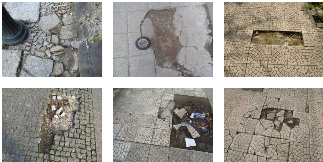
Figure 10: Sidewalks in Porto with various types of deformations. Photos by Fernando Fonseca, CTAC.
