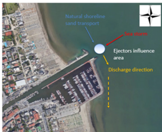
Fig. 10 - Aerial view of the harbor of Cervia. The project aims to evaluate the performances of the ejectors to restore the natural movement of sediments from North to South direction.
