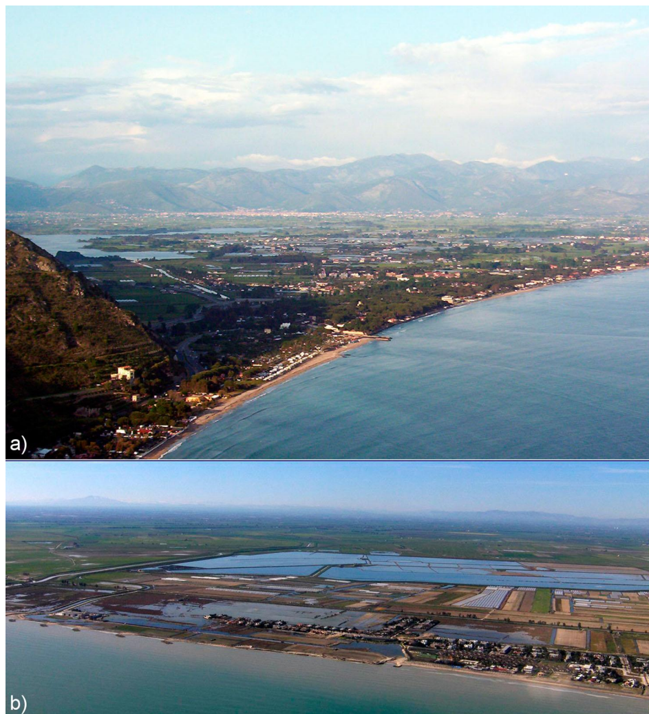
Figure 1. The Italian coastal areas are characterized by important human settlements that are sensitive to sea level rise: (a) the Fondi Plain, near Latina (Latium, Italy) is one of the 33 areas of the Italian coastal zones prone to marine flooding (Lambeck et al., 2011) (Photo G. Mastronuzzi, 2005); (b) the Mouth of Carapelle river, near Foggia (Apulia, Italy) with damaged wetlands after the sea-storms occurred on February/March 2009 (Photo by M. Caldara, 2009).
