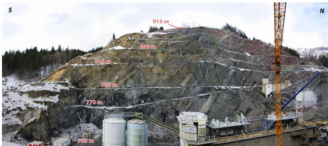
Fig. 1 Panoramic view of the quarry site where bench elevation is indicated
