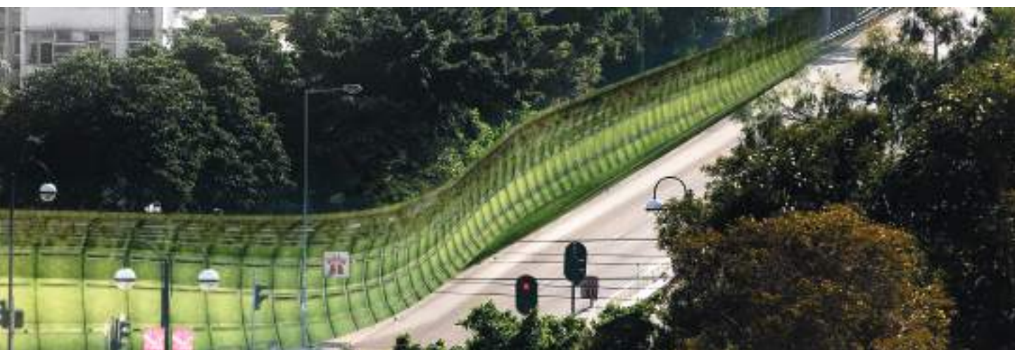
Figure 5.8. Green noise barrier, (©ESKYIU). ( http://eskyiu.com/linear-landscapes/ )
