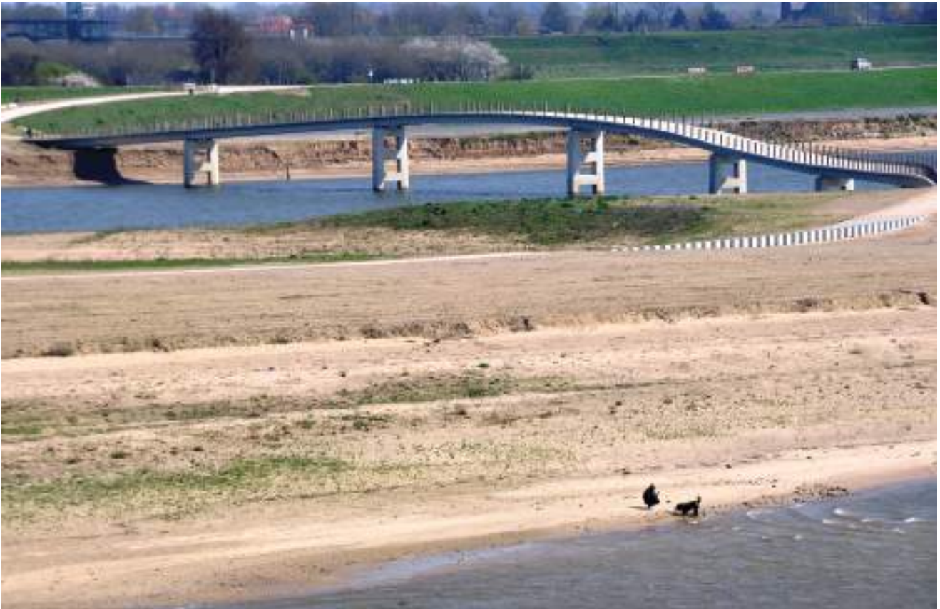
Figure 7.6. Part of the Room for the Waal project area ( https://www.flickr.com/photos/maldeno/26306868451/in/photostream/ )
