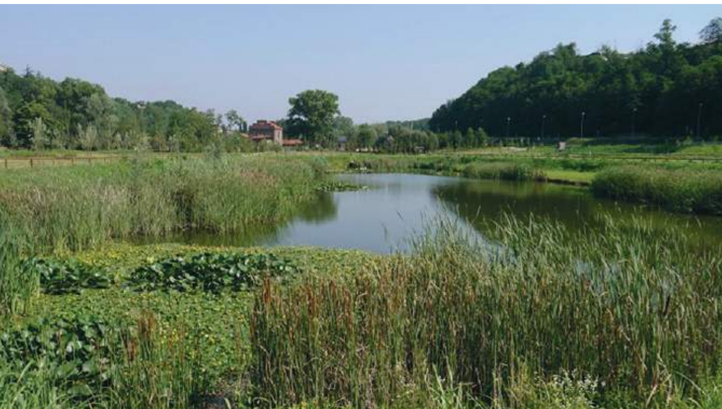
Figure 5.17. Constructed wetland in Gorla Maggiore, Italy ( https://oppla.eu/casestudy/17252 )
