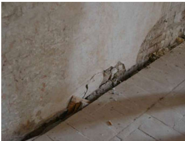
Figure 6: Detachment between the floor and the East wall of the Giulio II Hall after the Emilia earthquake.
