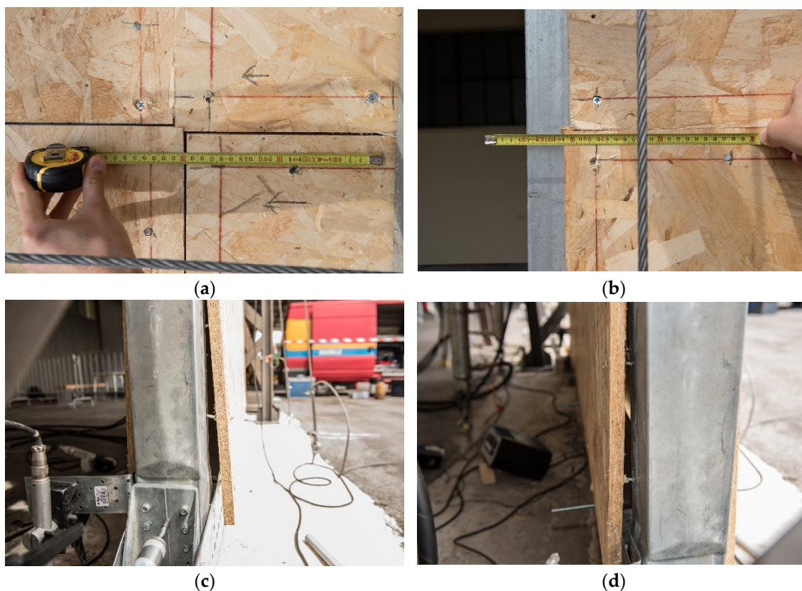
Figure 9. Details of failures evidenced in test: (a,b) relative slip between panels; (c,d) withdrawal of self-drilling screws and crushing of the steel column.
