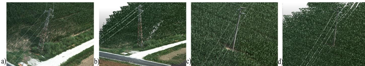
Figure 1. Examples of image-based 3D reconstruction of power line corridors. Starting from helicopter-based imagery (a, c), dense point clouds of cables, transmission towers, pylons and surrounding environment can be generated (b, d).
