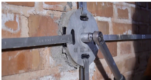
Figure 14. Tightening of a threaded bar [54].
