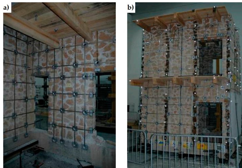
Figure 9. An example of reinforcement with the CAM system: 2:3-scale model for testing on a shaking table [48]: (a) internal view; (b) external view.
