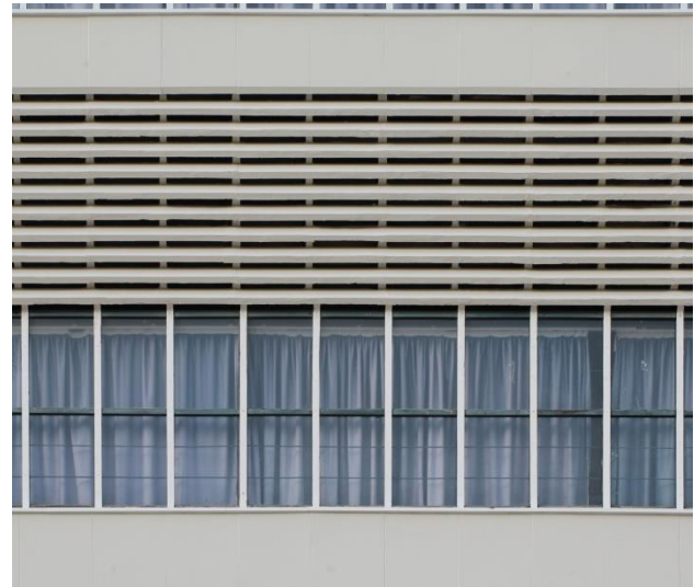
Figure 5. Current image of fixtures towards the street.
