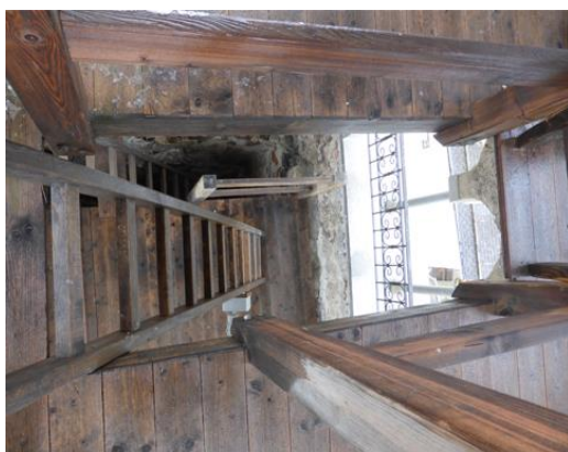
Figure 2. View of inside from A floor
