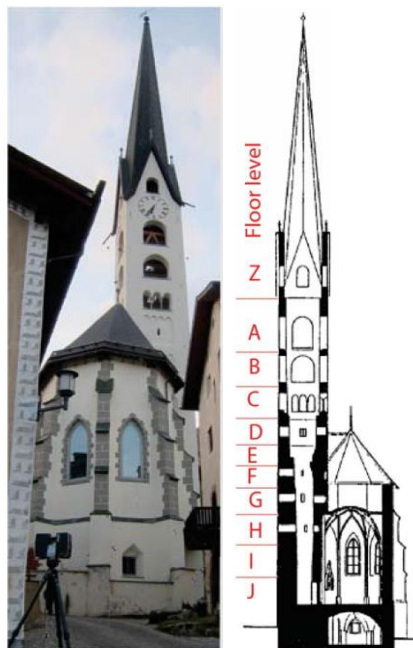
Figure 1. Left: San Luzi church bell tower. Right: cross section of the bell tower with its floor plan
