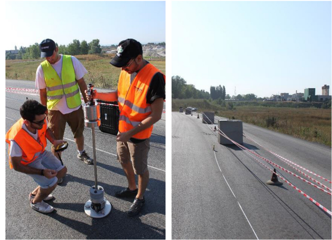
Fig. 8. LWD test (left) and trial field (right).
