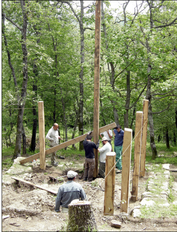
Fig. 4 – The vertical woodwork of the house.
