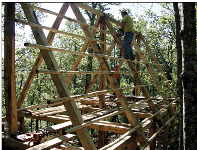
Fig. 7 – The roof's purlins.
