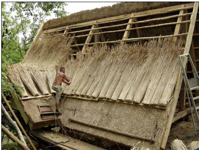
Fig. 9 – Roof material: water reeds.
