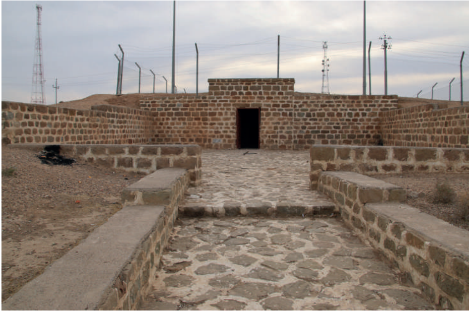
Fig. 4 - The entrance to the Parthian-period tomb of Sarqala created when the site was musealised. Photo D. Andreucci – MiSAK 2021.
