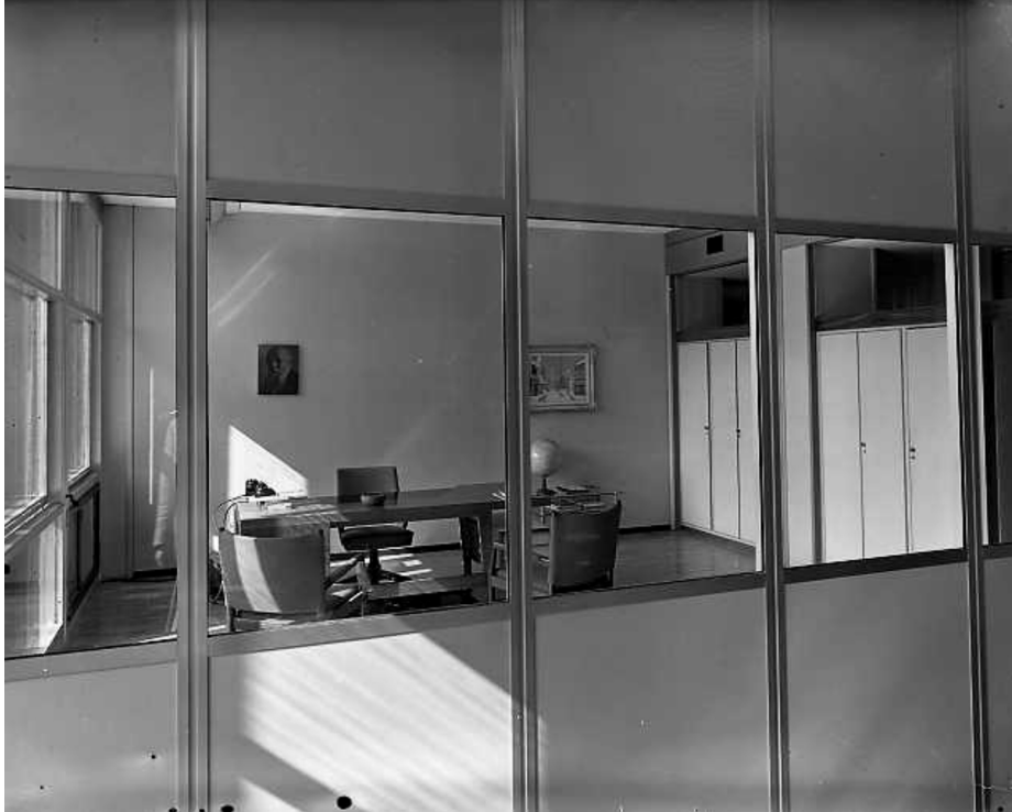
Fig. 20. The “Anacoustic” removable partition walls. In the background, one of the offices and the succession between doors and closets (source: Associazione Archivio Storico Olivetti, Ivrea - Italy, Faldone 26)
