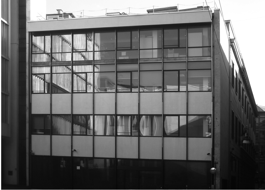
Fig. 12. The lower height of the wing near Palazzo Clerici , similar to the surrounding context – (photography: Federico Cinti – elaboration: Carlo Costantino)
