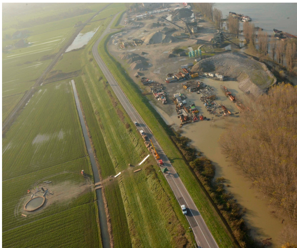
Figure 4. An aerial view of the largest historical sand boil (#36(2)) in Boretto, during the November 2014 reactivation. In the background, note saturated areas landward, due to underseepage. (Image courtesy of the Italian Firefighters Corps, Vigili del Fuoco).
