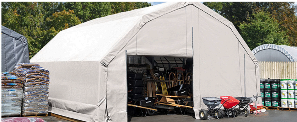
Fig. 2. A picture of an OSW used as a material storage place at a construction site.
