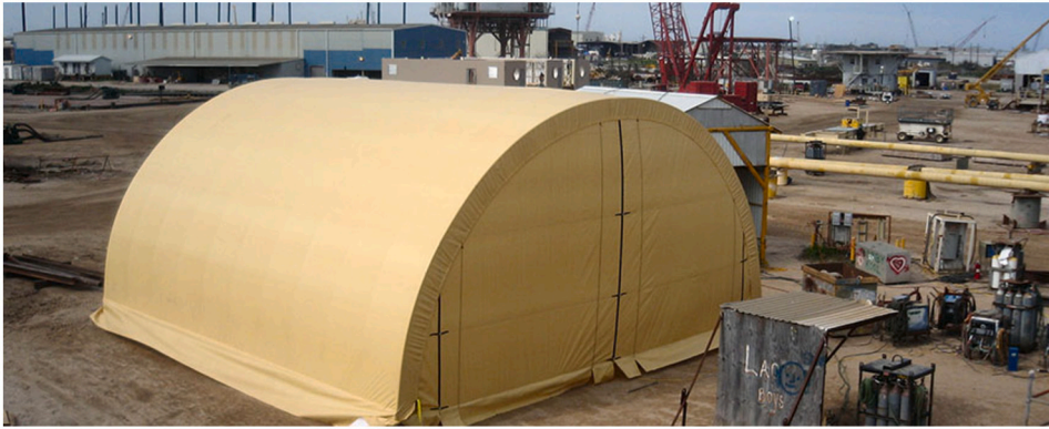
Fig. 1. A picture of an OSW at a construction site.
