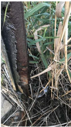
Fig. 11 a) Deterioration of the fibreglass layer that initially wrapped metallic tubes; b) corrosion of metallic framework near the base (two joined flanked tubes and their connection to the basement can be seen); c) rising of the level of ground water during the rainiest periods (courtesy of Antonello Zoffoli).
