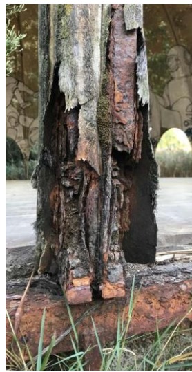
Fig. 11 a) Deterioration of the fibreglass layer that initially wrapped metallic tubes; b) corrosion of metallic framework near the base (two joined flanked tubes and their connection to the basement can be seen); c) rising of the level of ground water during the rainiest periods (courtesy of Antonello Zoffoli).
