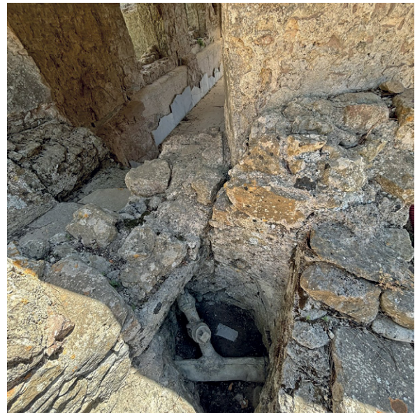
Fig. 5. Section of the aqueduct connected to the frigidarium and a lead fistula in situ , view from the southwest (photo by C. Lamanna, 2024).
