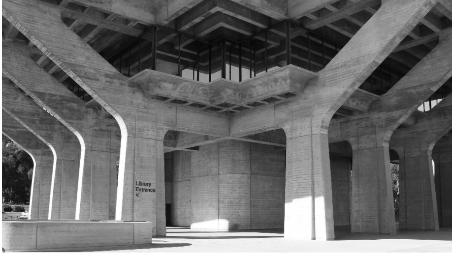
Fig. 10. Detail of massive pillars in concrete (photo by Caterina Morganti, 2020).
