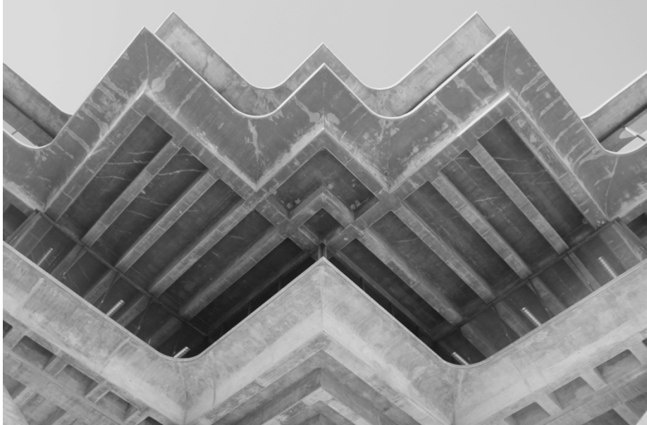
Fig. 13. Detail of interlacement of beams (photo by Caterina Morganti, 2020).
