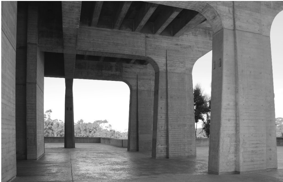
Fig. 11. Detail of massive pillars in concrete (photo by Caterina Morganti, 2020).
