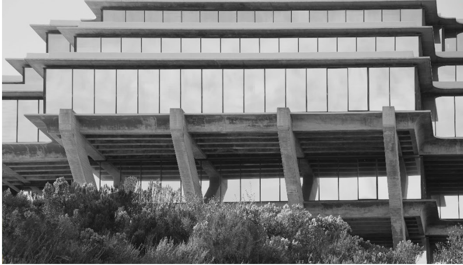
Fig. 8. Detail of glazing (photo by Caterina Morganti, 2020).
