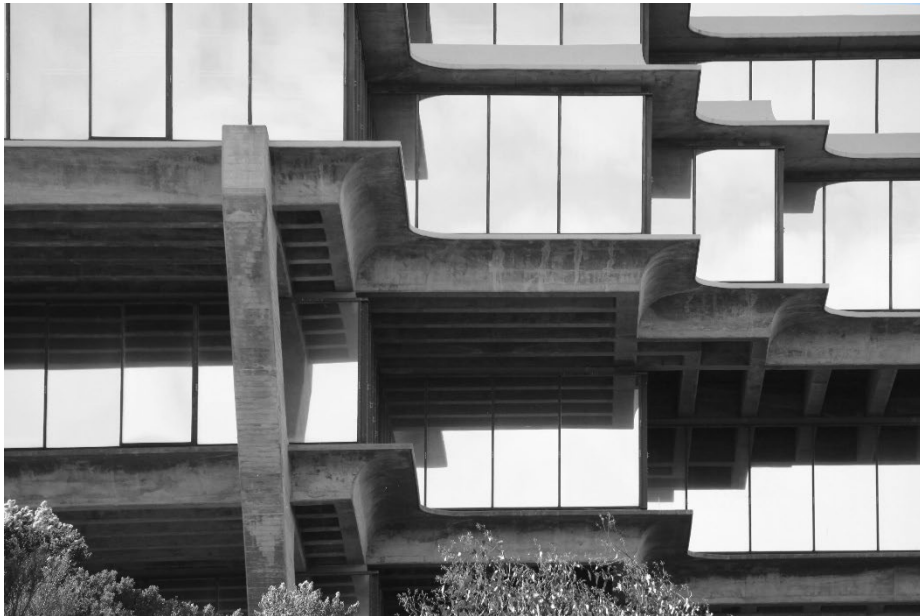
Fig. 9. Detail of glazing (photo by Caterina Morganti, 2020).
