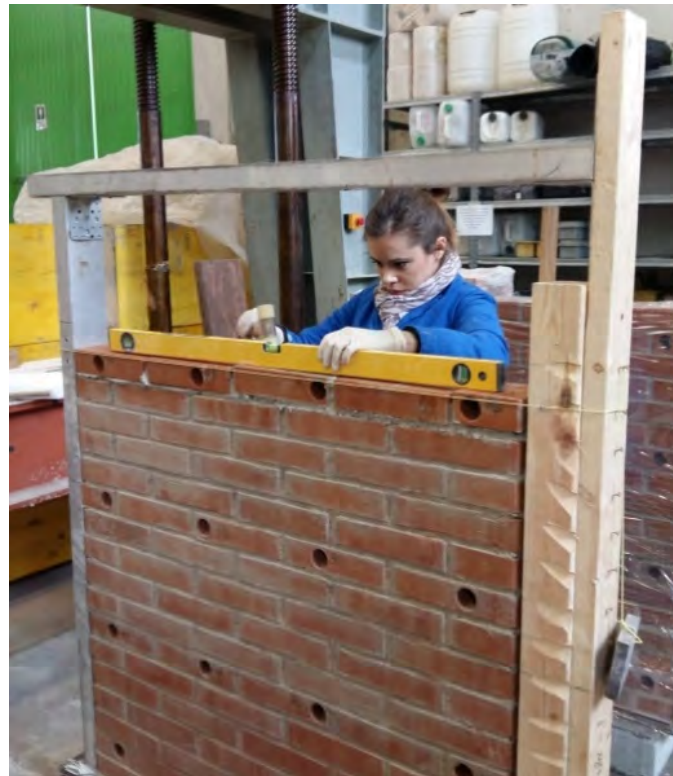
Figure 18. Equipment used for the correct laying of bricks.
