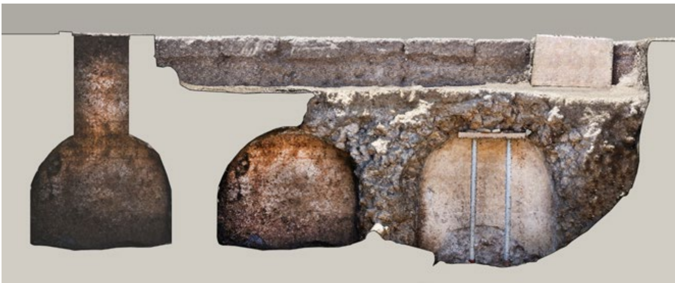
Fig. 8. First corridors of the large cistern in the forecourt of the sanctuary of Apollo (F. Giannella).
